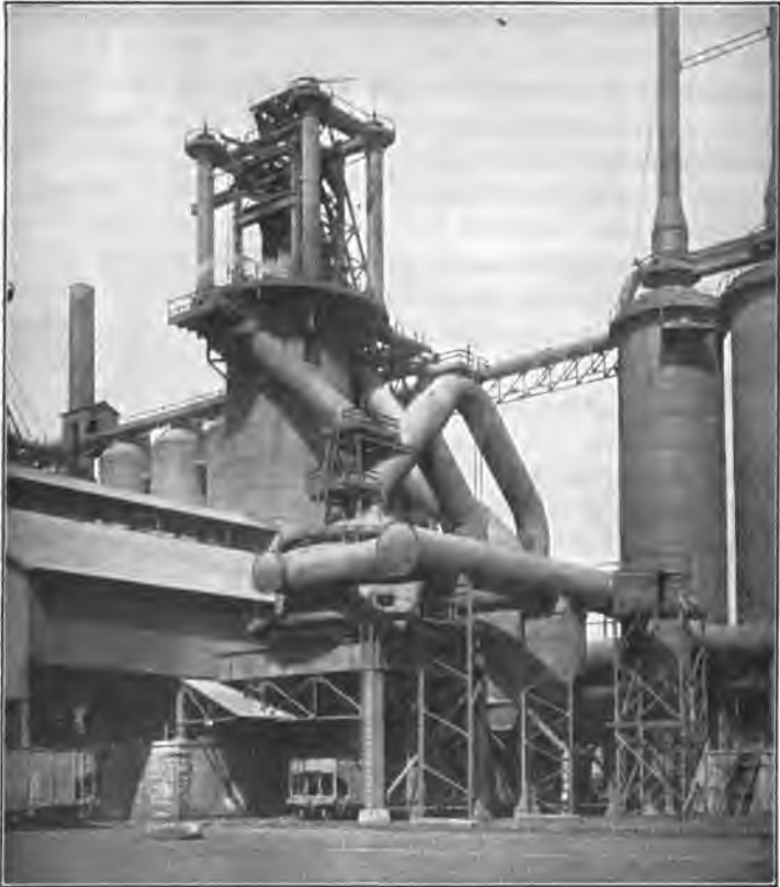
FIG. 94.—A blast furnace for reducing iron ores. The "stoves" seen at either side heat the air for the blast.
